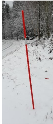
Figure 13 Snow pole marking the edge of the road (poles are located some distance outside the drivable area).
